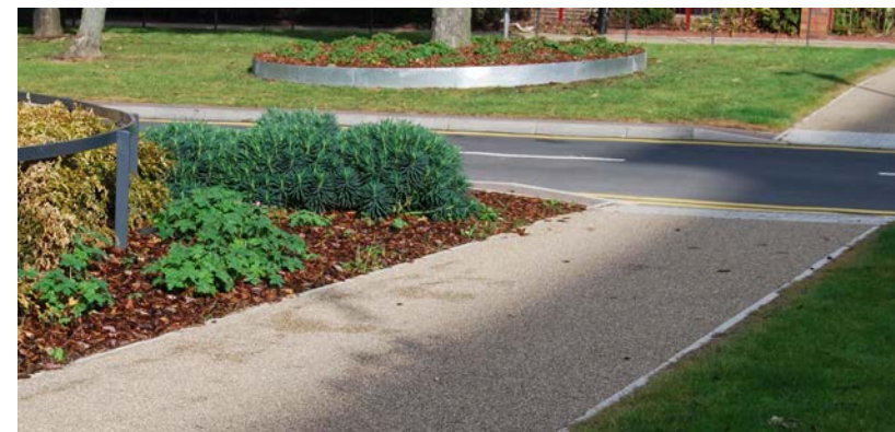
Pavement in a buff colouring such as Tarmac Ultracoloured asphalt
